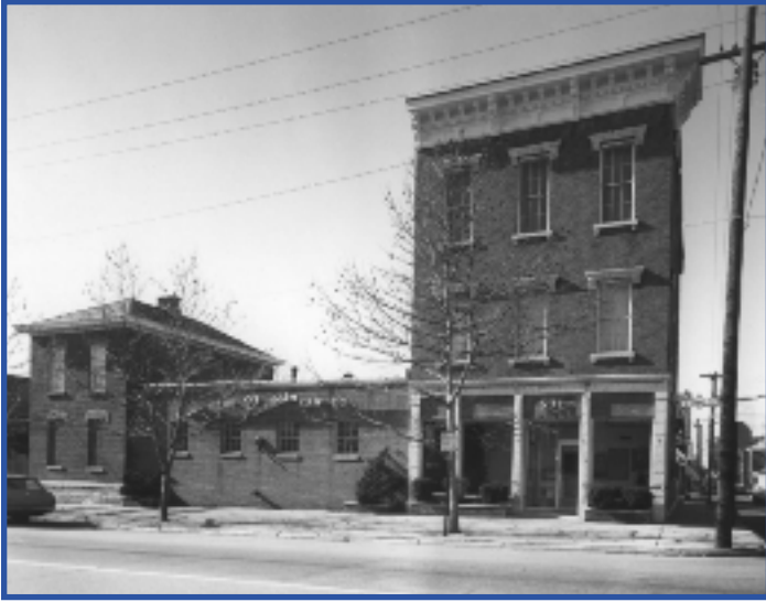
Peerless building in German Village
